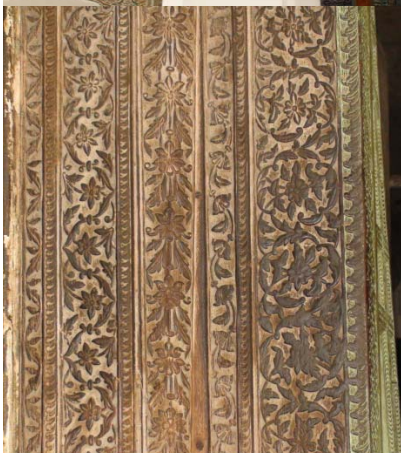
Fig.4.Pillar and ceiling of veranda, Fig.5. Filigree, entrance frame door,
