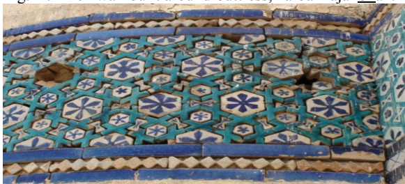
Fig.22. Kashīkāri, façade buttness, Layyah.
