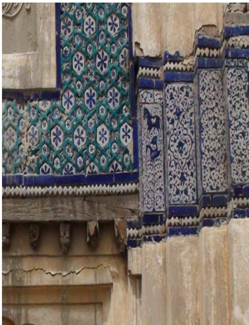
Fig.27. Ornamental band, right-side of the four-foil pilaster, Southern façade, glazed tile, Darbār Rājan Shāh, Karor La'leason, Layyah.
