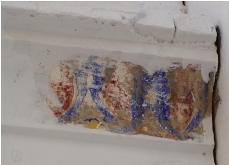
Fig.31. Fresco work being white washed, DarbārRājanShāh, KarorLa‘lEason, Layyah.
