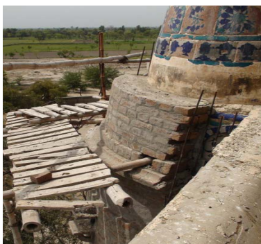
Fig.21. Brick wall built around buttness, DarbārRājanShāh. KarorLa‘l Eason, Layyah.
