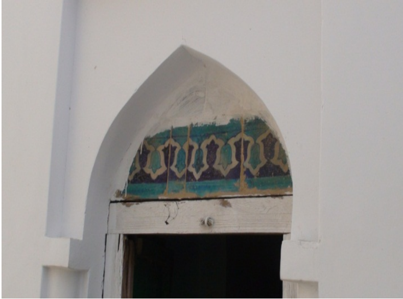
Fig.30. Glazed tile-work being white washed, DarbārRājanShāh, KarorLa‘lEason, Layyah.
