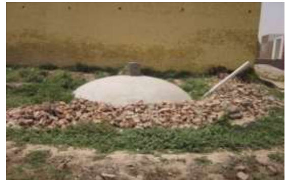
Fig. 20 Biogas plant in Miani Mallah Source: Photograph by the Authors, 2011
