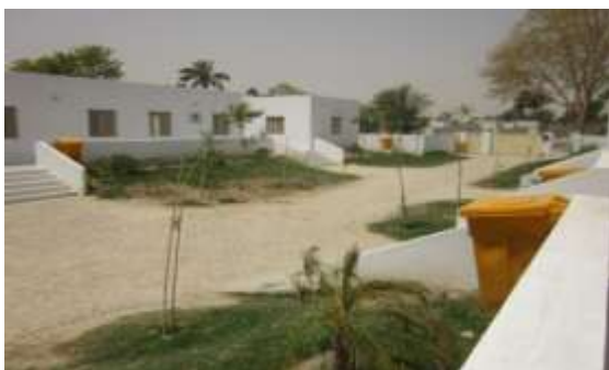
Fig. 17 Primary School in Miani Mallah Source: Photograph by the Authors, 2011
