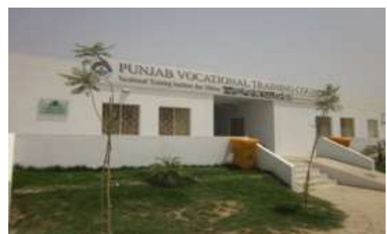
Fig. 21 Vocational training institute in Miani Mallah Source: Photograph by the Authors, 2011
