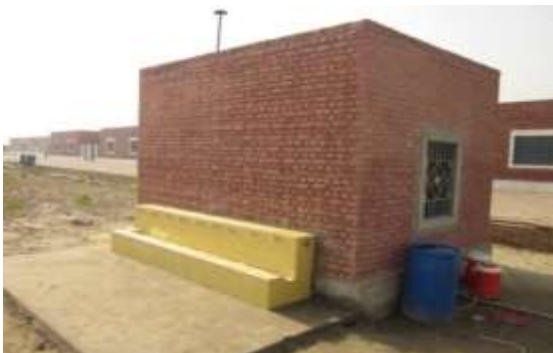
Fig. 8 Water filtration plant in Noor Ghazi Source: Photograph by the Authors, 2011
