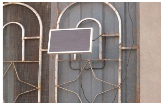
Fig. 12 Solar Cells outside houses in Noor Ghazi Source: Photograph by the Authors, 2011
