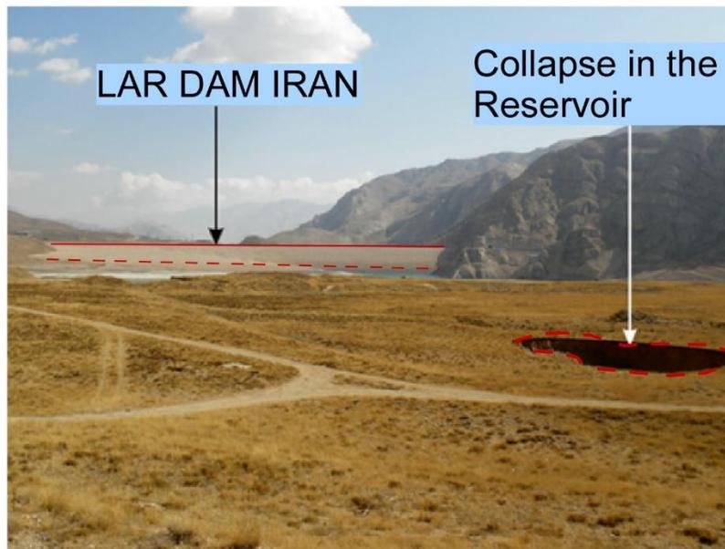
Figure 1. Location of Lar Dam and development of collapse in reservoir due to limestone karstification [modified after Kh. Fegghi [18]
