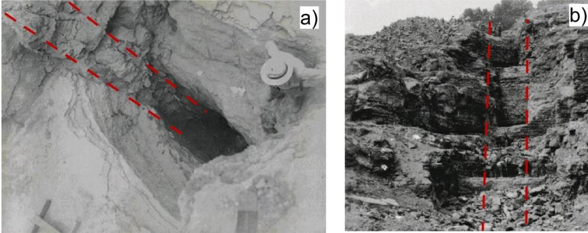
**Figure 2. Location of the extensive seepage points in the Central Hill Dam, a) vertical joint, b) location of the damaged cutoff wall due to erosion, modified after L. Adcock [10].**
