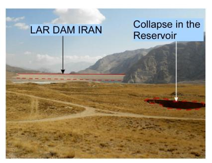
Figure 1. Location of Lar Dam and development of collapse in reservoir due to limestone karstification [modified after Kh. Feghhi [18]
