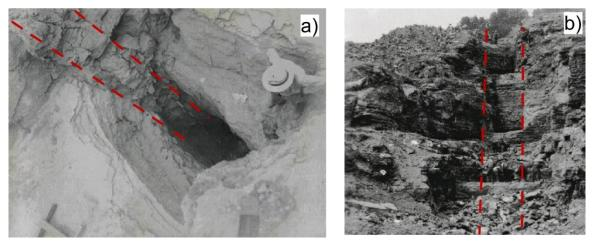
Figure 2. Location of the extensive seepage points in the Central Hill Dam, a) vertical joint, b) location of the damaged cutoff wall due to erosion, modified after L. Adcock [10].
