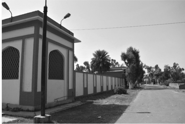
Figure 8. View of the southern wall around the tomb
