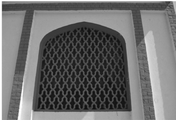
Figure 7. Details of terracotta lattice or jāli work on the façade of the eastern walls Source: Photograph May 6, 2023
